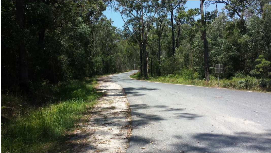
Figure 6-2 Looking east from site access
