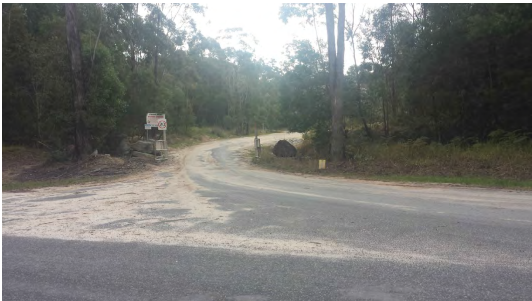
Figure 1 Site Access Road and Gate
