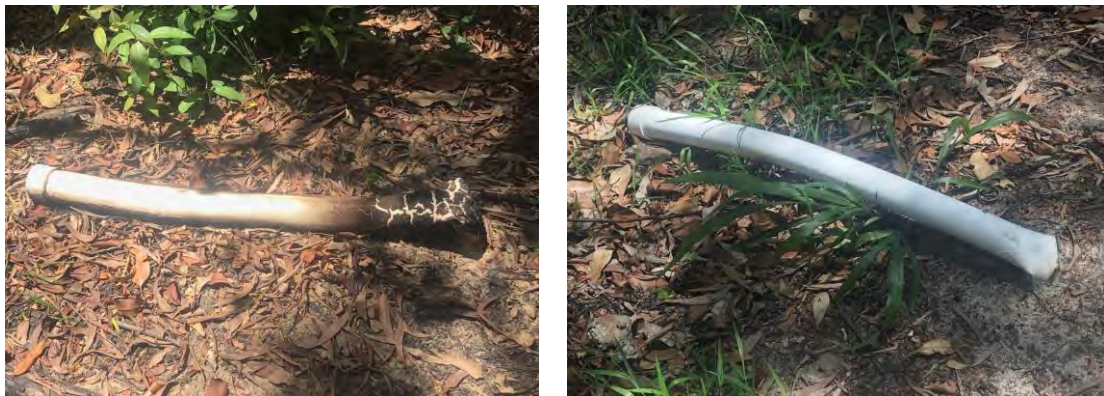
Figure 6-2 Bushfire damaged groundwater wells
