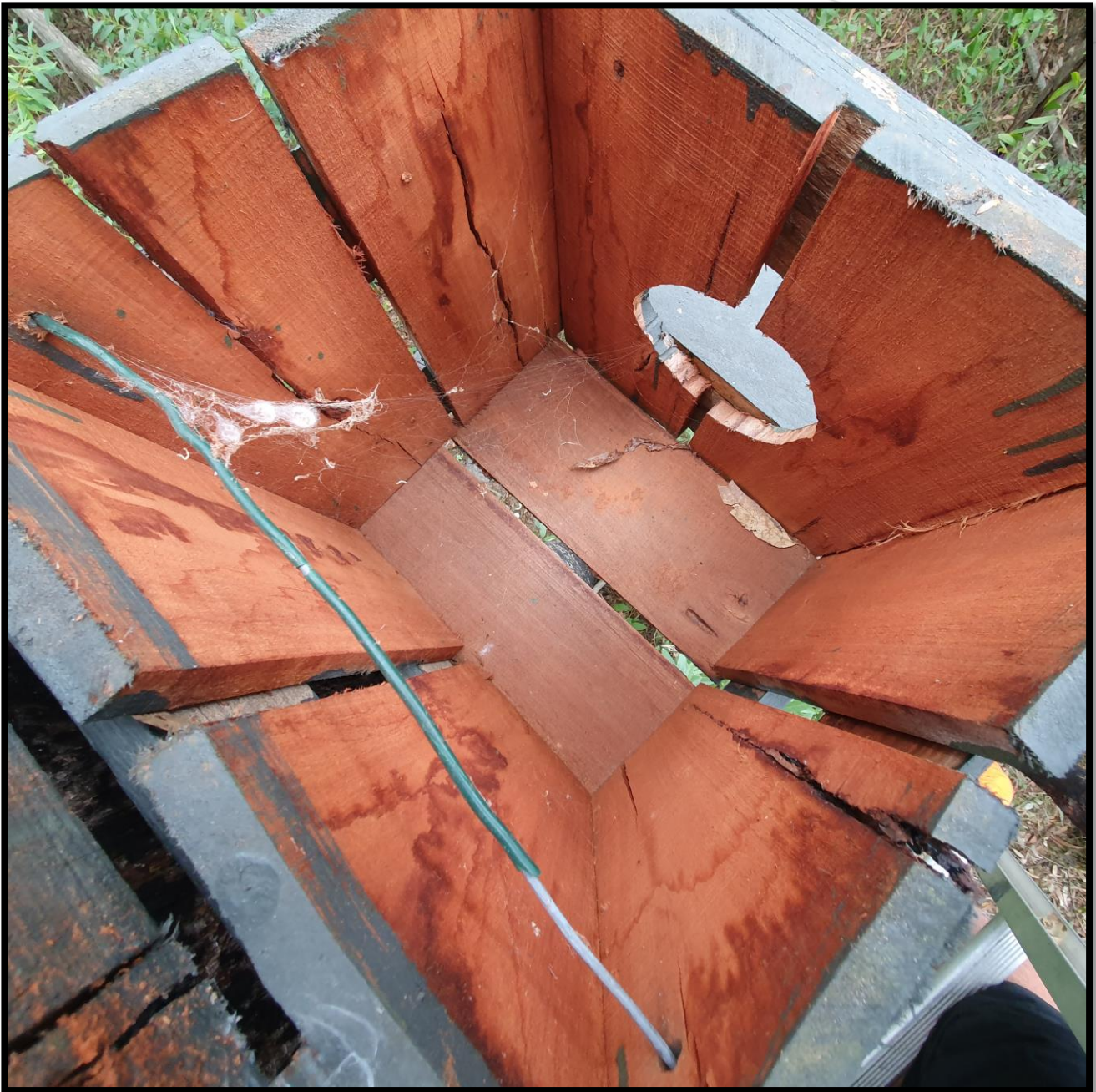
Plate 4-1. Example of nest box identified for “cladding” to reduce the gaps that allow sunlight, wind and rain egress.
